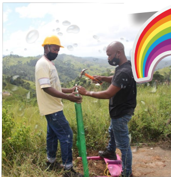
Tippy Taps being constructed by Thanda maintenance team near roadside bus stop.
